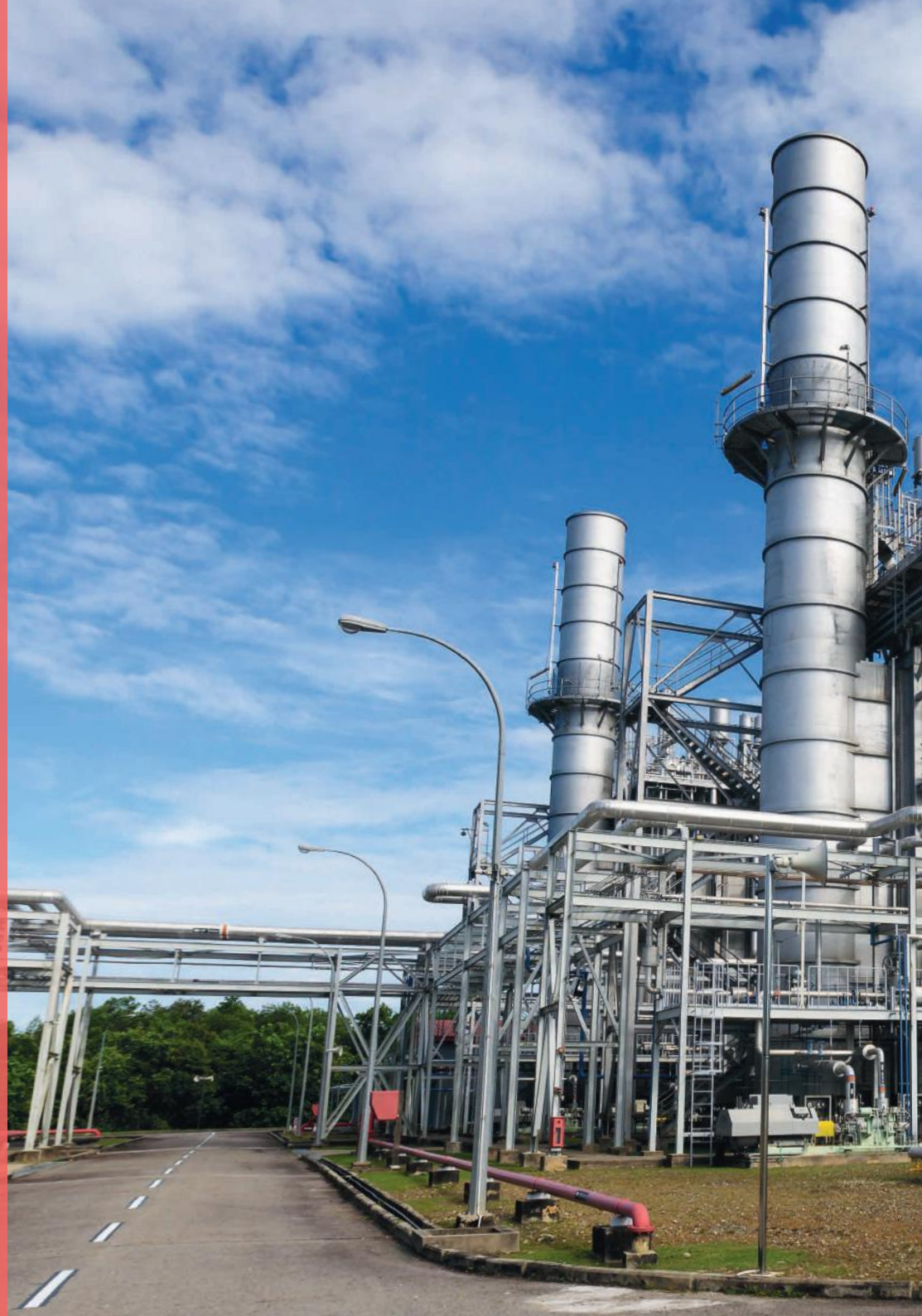
Combined-cycle Gas Power Station, Bukit Panggal
