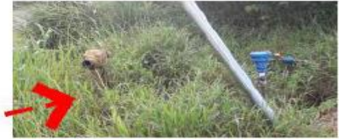
EXISTING FIRE HYDRANT WATER METER
