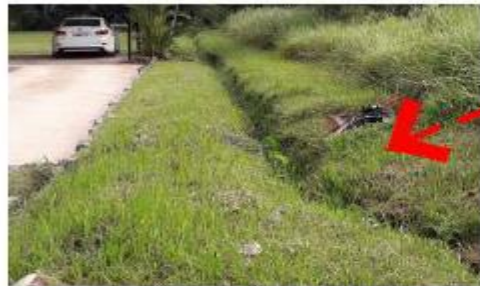
EXISTING EARTH DRAIN
