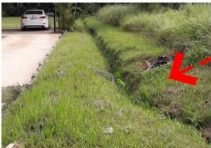
EXISTING EARTH DRAIN
